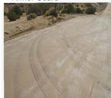
12) Finished road is Hard as a rock
