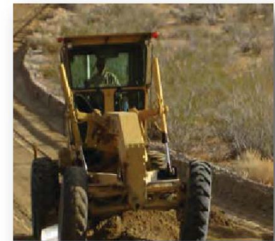
6) Wind row soil to the center of the road
