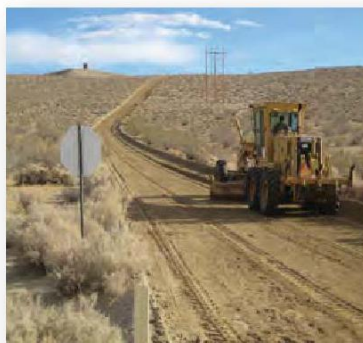
8) Blade soil at center to grade.
