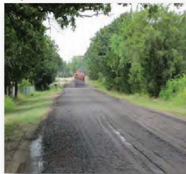
5) Apply Armor Guard solution to disturbed road
