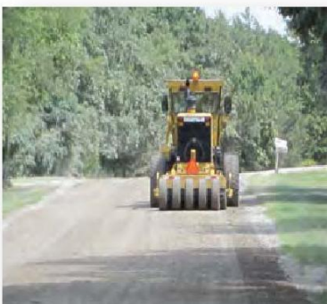
10) Roll area to 95% compaction
